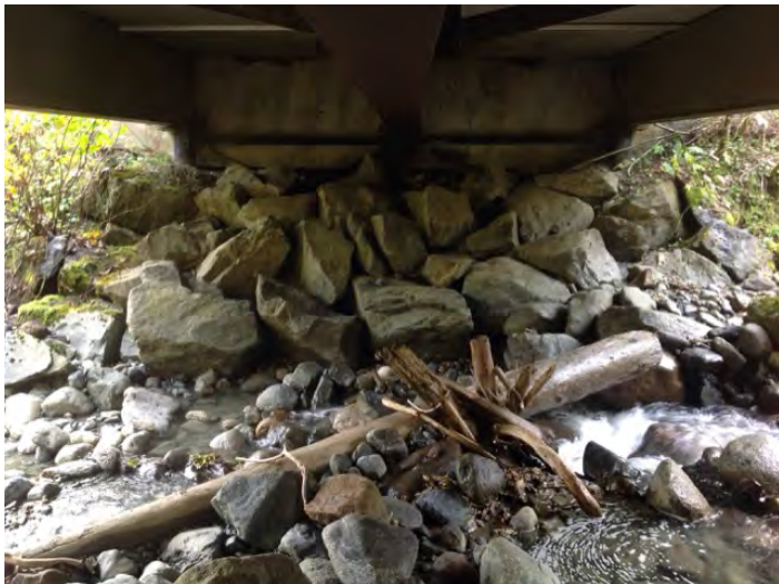
Right Bank Abutment when facing downstream
