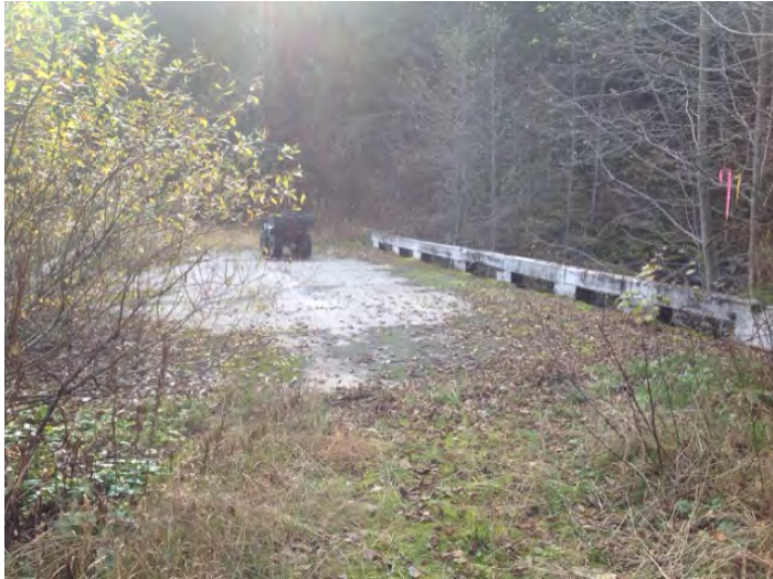
Approach from Left Bank when facing downstream
