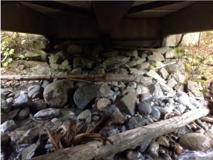
Left Bank Abutment when facing downstream
